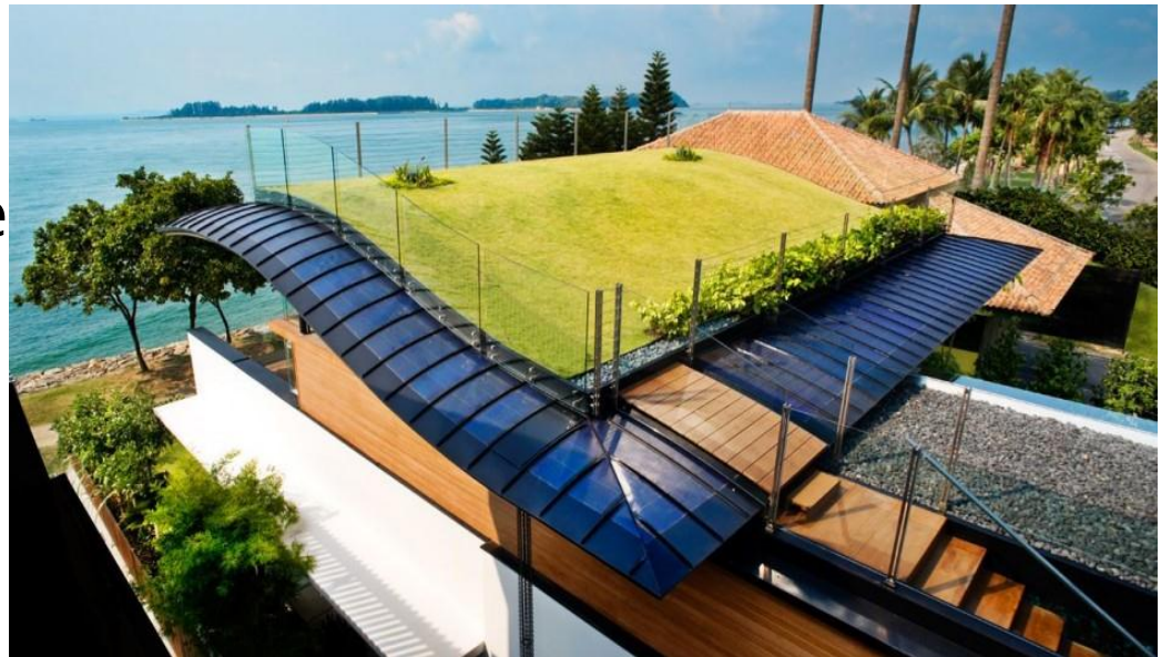
Angled view of the roof.
