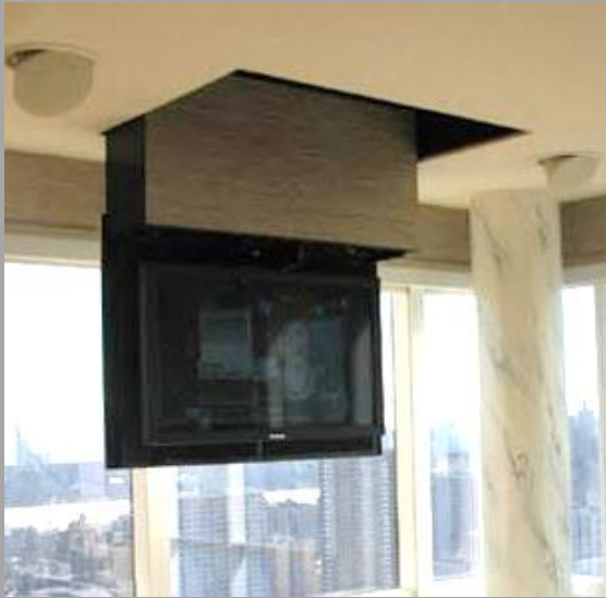
CUSTOM BUILT DROP DOWN TELEVISION
