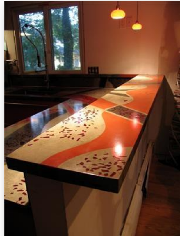
a poured slab with recycled glass chips
